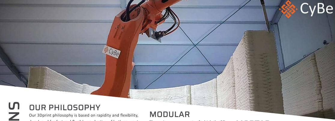
Our 3Dprint philosophy is based on rapidity and flexibility, developed for fast and flexible production of both pre-cast and on-site printed elements. Due to this philosophy, the size of a building is not the main factor - a larger object such as a building can be constructed very fast by connecting the different elements without the need for a bigger printer. Due to easy use and rapid curing, multiple elements - walls - can be printed in one day.
