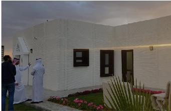
3D printed homes are set to become mass production solutions in the middle east. Thanks to a world-first project in Saudi Arabia, with CCC testing the technology, this 80 m<sup>2</sup> single bedroom house consists of 48 elements. 27 walls and 21 parapets which we have printed on-site in only one week.
