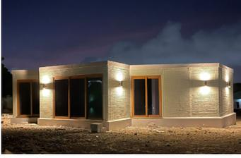
Our team printed together with the help of our partner Betonindustrie Brievengat in Curaçao the first 3D printed building on the island. During the on-site training the walls of the Office building were printed off-site and afterwards transported to the final location. The building consists of 13 printed walls, printed in only 7 days.
