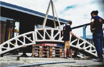
In cooperation with the Antea Group we produced a bridge that is built out of 3 segments. It only took 45 minutes to fabricate every piece. Also we could produce all the elements without relocating our crawler. The total printing time was 2 hours and 15 minutes. After the hardening process the elements were shipped towards their final destination.
