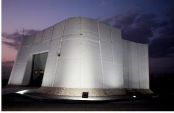
In order for DEWA, CyBe has produced the R&D Laboratory. This building is the 1<sup>st</sup> approved 3D printed building in the UAE within the municipality of Dubai. CyBe was responsible for the engineering and construction of the building. The project was delivered in the second quarter of 2017.
